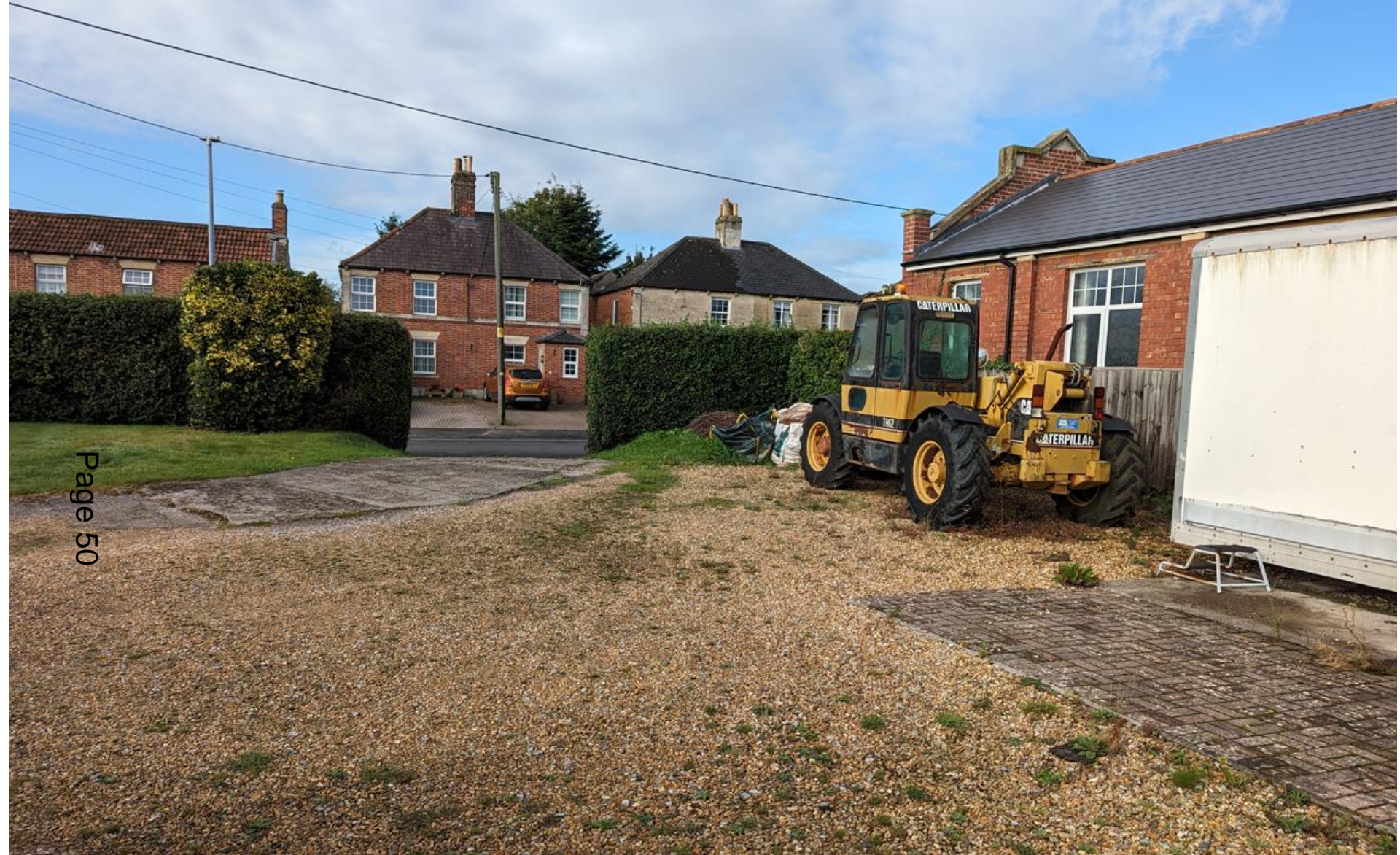
View from within the site and proposed access looking back to Woodmarsh
