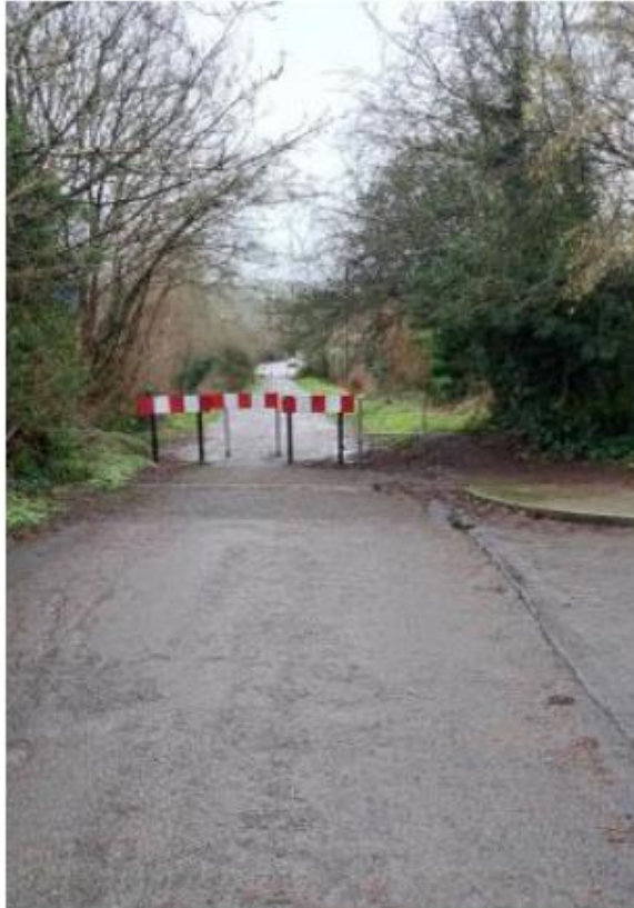
The pedestrianised footway leading to Apsley Close in Trowbridge
